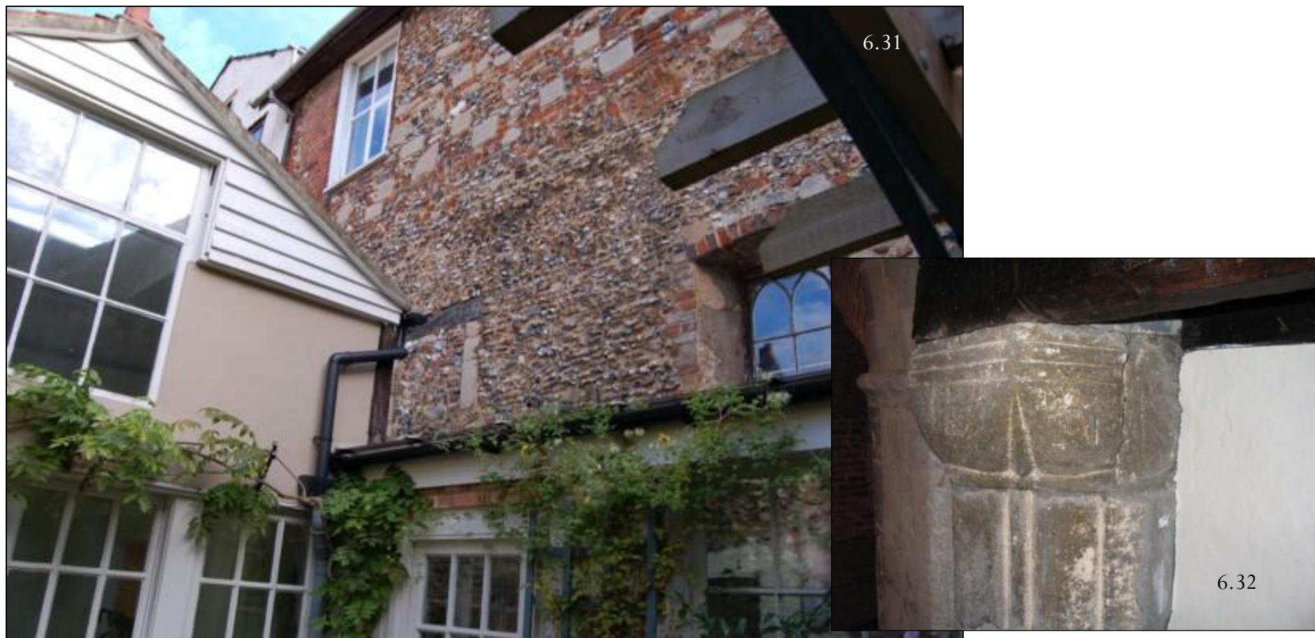
Figure 6.31 Rear wall of 25 Hatter Street, photographed from the south-west. A door or window is visible at first floor height. The change from flint rubble to brick occurs at a height of 5.20m. Figure 6.32 Jamb from a fireplace which was removed from this house in the 19 th century and which is now in Moyse's Hall Museum.
