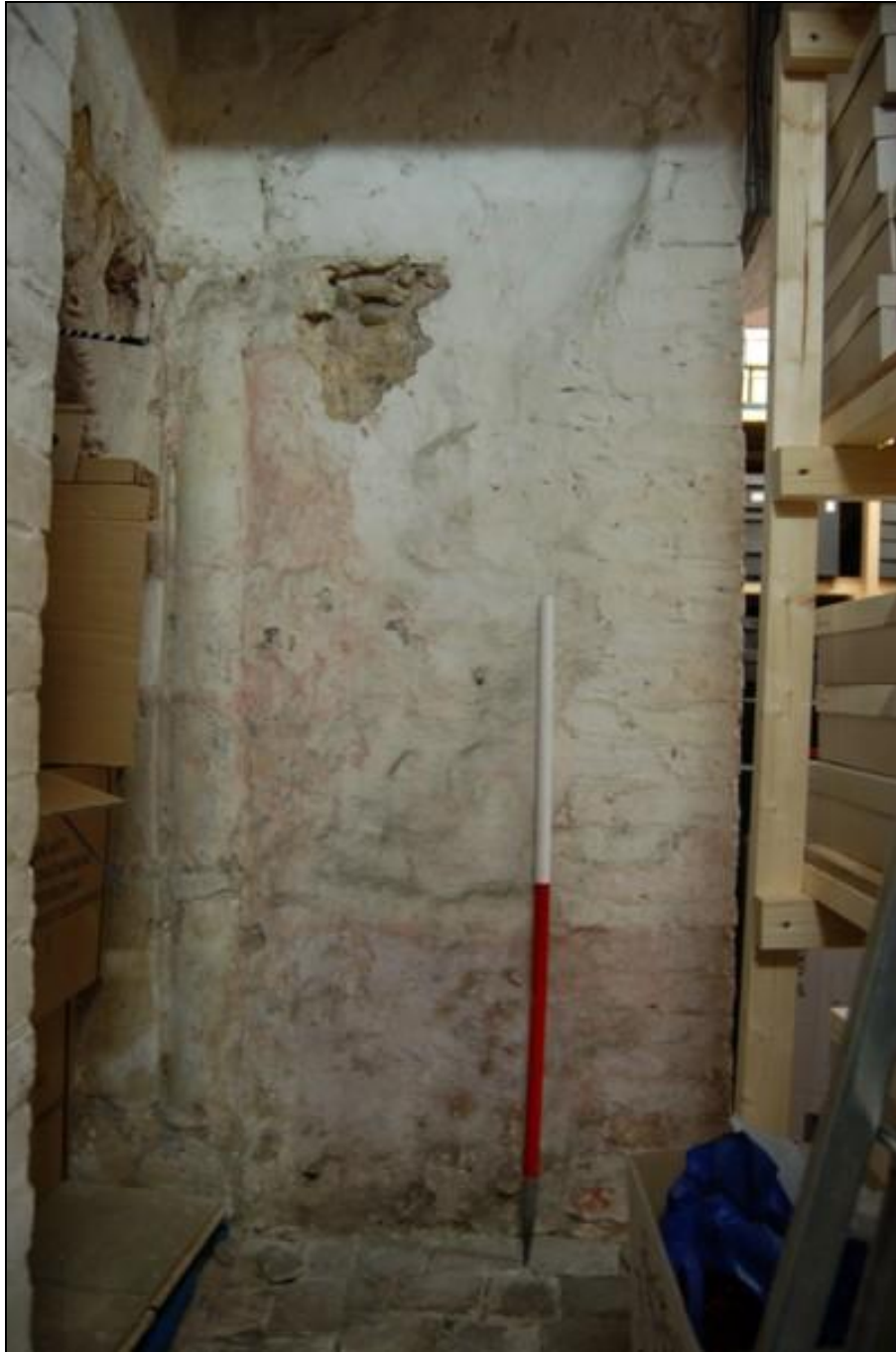
Figure 6.46 9B the Traverse, fragments of stonework. Photographed from the south. The rubble behind the stone lends weight to the hypothesis that this is in situ . However, the pillar is disjointed and the base of it appears to be an upside down capital – although this latter feature is not unknown in Romanesque work. The scale is 1m long.
