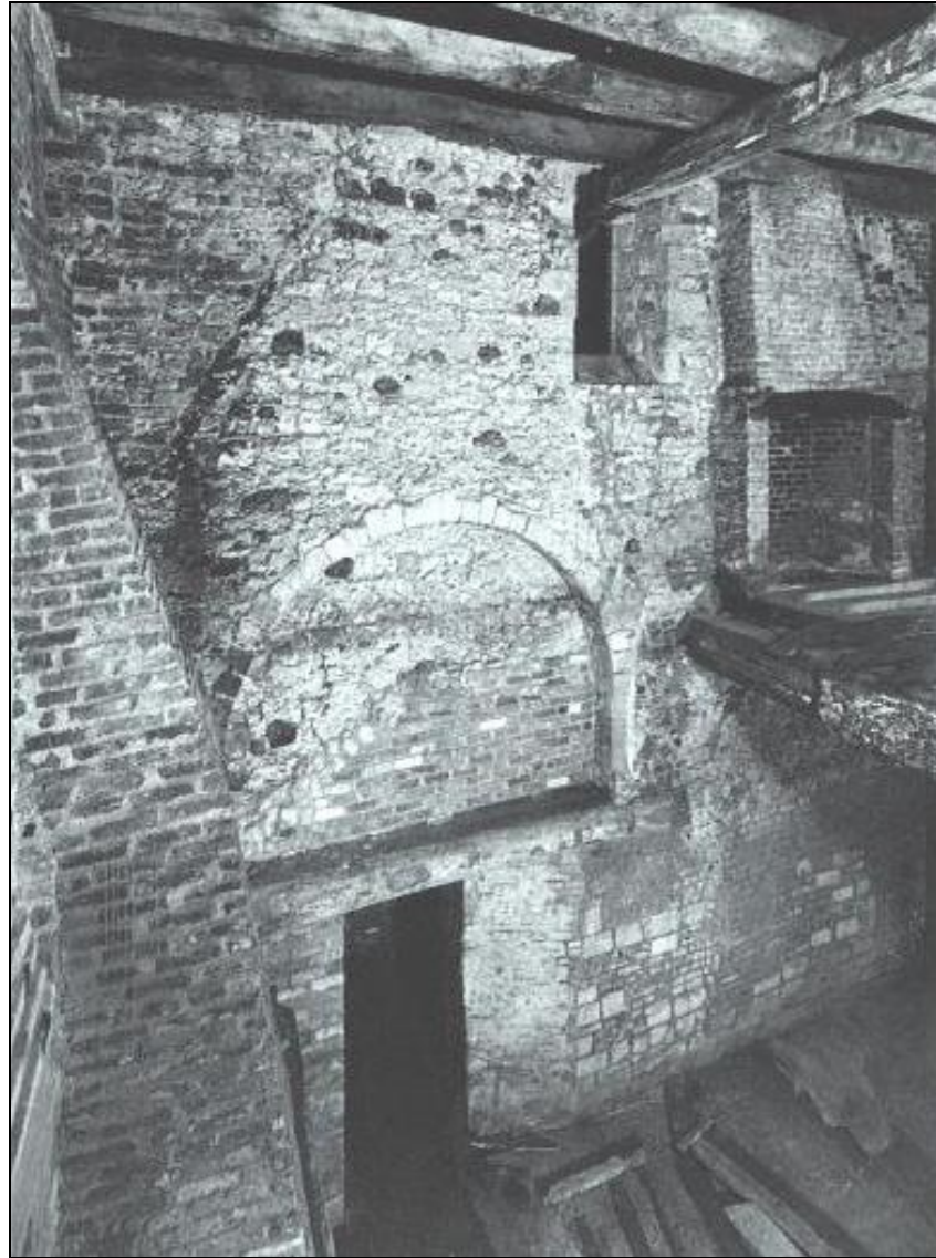
Figure 2.6 The south gable of 28-32 King Street, King's Lynn, now demolished. The wall with the arcade dates to c. 1200 (Taylor and Richmond 1987: plate III).
