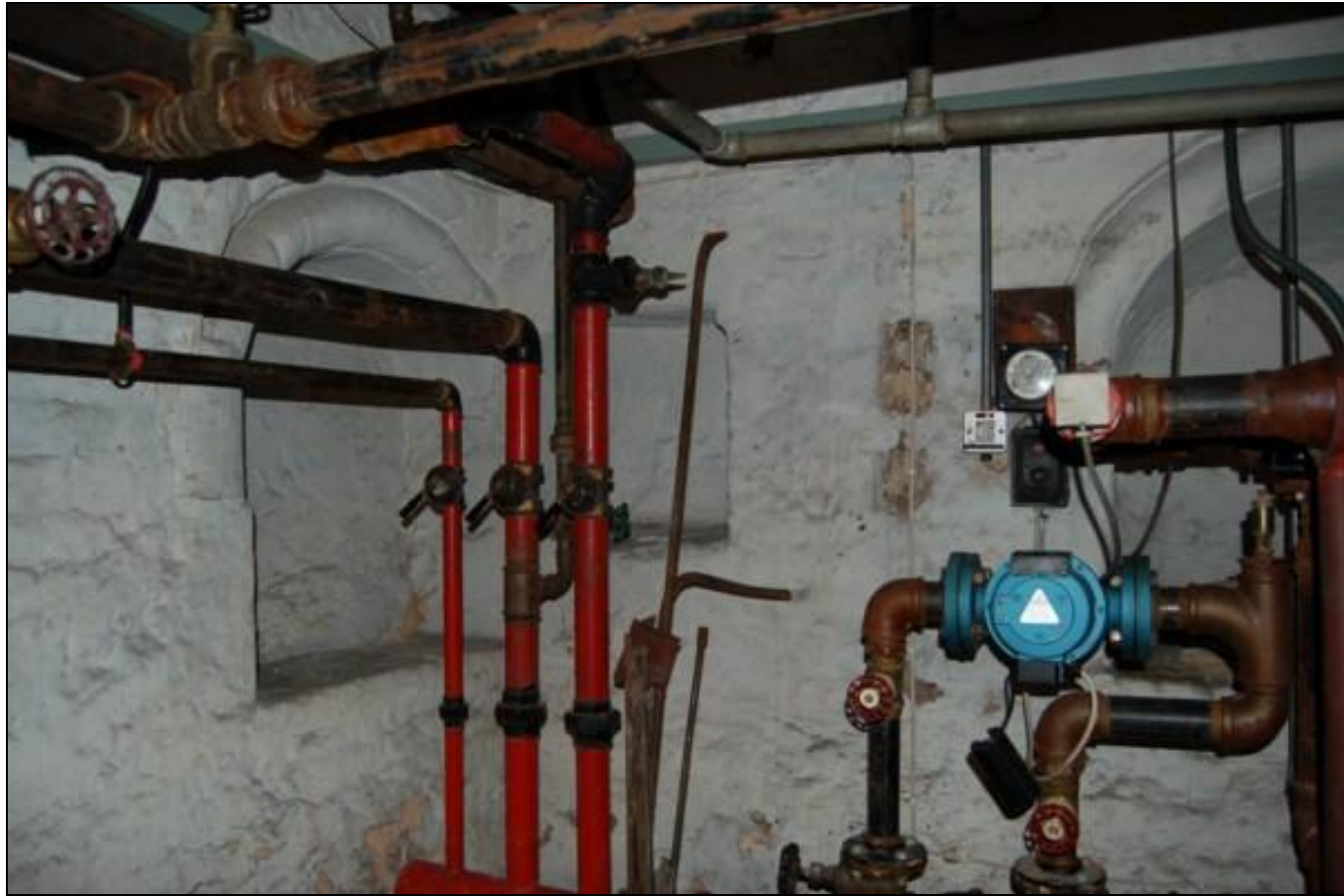
Figure 6.44: Features within 111 Northgate Street, photographed from the north. The boiler system was an obstacle to recording.
