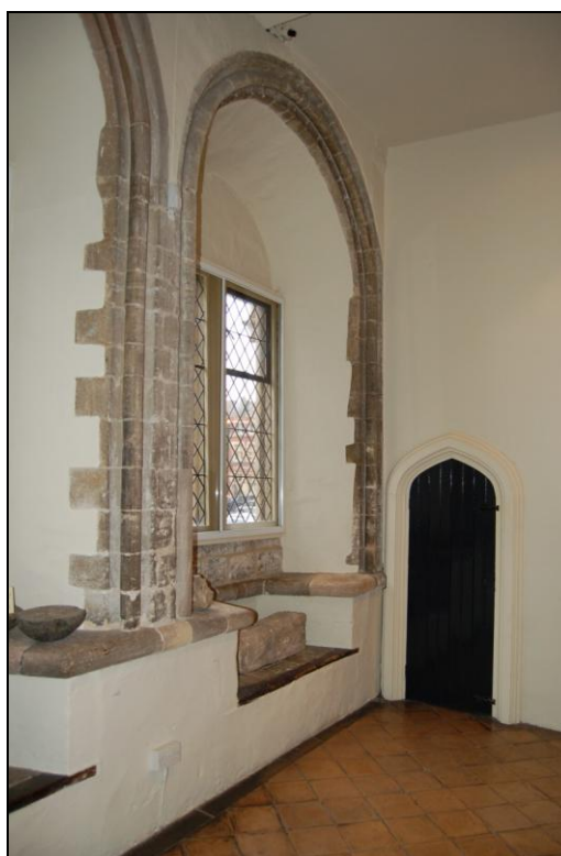
Figure 6.18 Window seats in the first floor room of the eastern part of Moyse's hall, facing south onto the market place.
