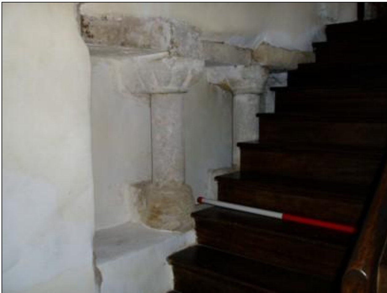
Figure 6.42 Stonework in the party wall between 63 Whiting Street and 30 College Lane., photographed from the south.
