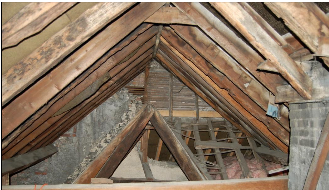
Figure 6.30b: Roof structures within 7, Hatter Street (facing north).
