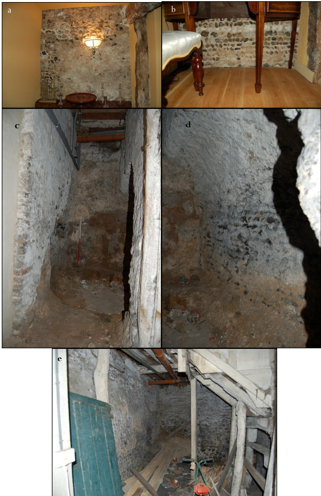
Figure 6.37 Walls in the basement of 33-34 Churchgate Street. a and b) at first floor level in 33, photographed from the south, c) an opening cut through the eastern continuation of the same wall, showing archaeological deposits, in number 34, d) northern return of the wall, e) eastern side of the wall. See Figure 38 for a plan of these features.
