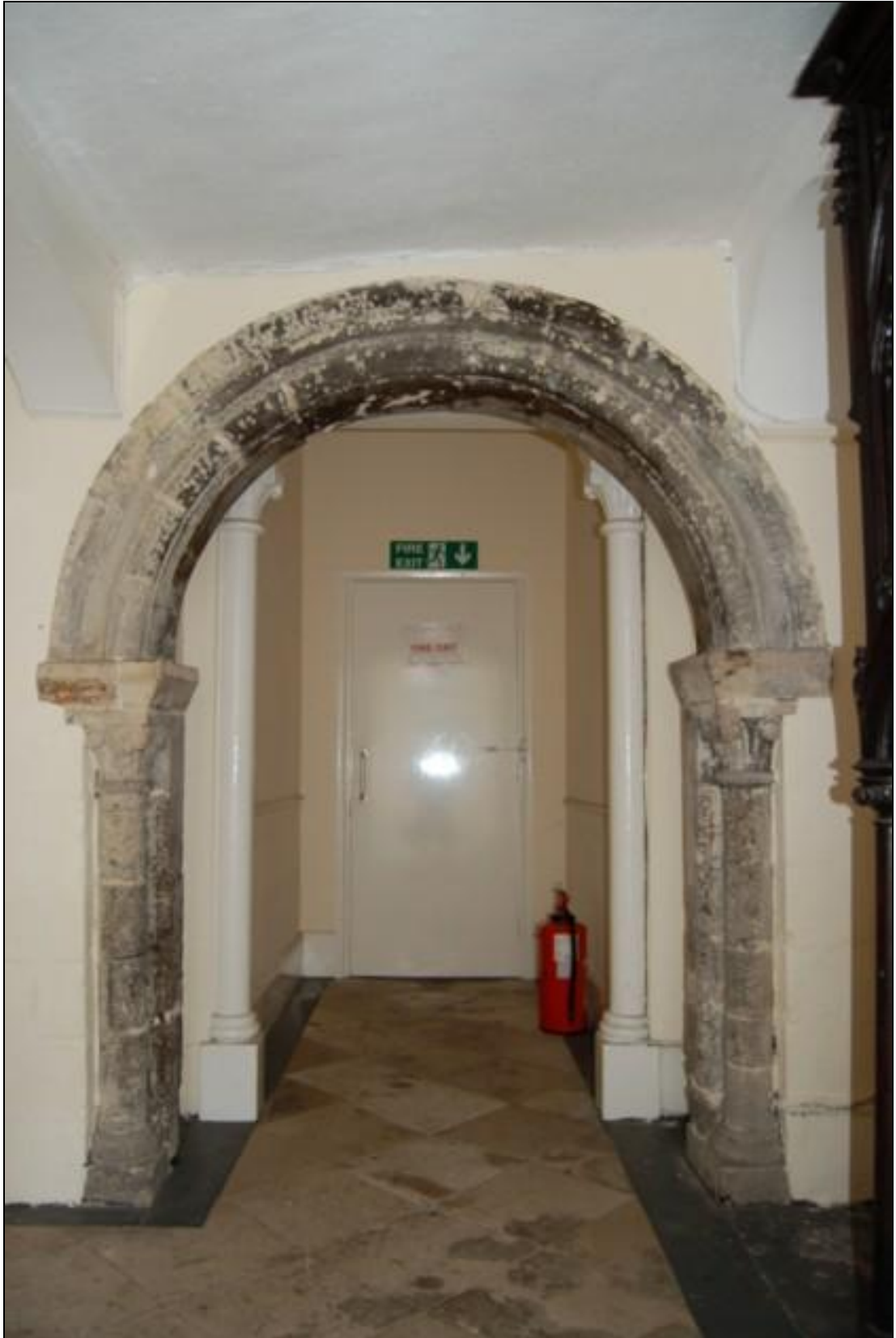
Figure 6.23 The Romanesque doorway within 79 Guildhall Street, photographed from the west. The arch looks to have been repaired.
