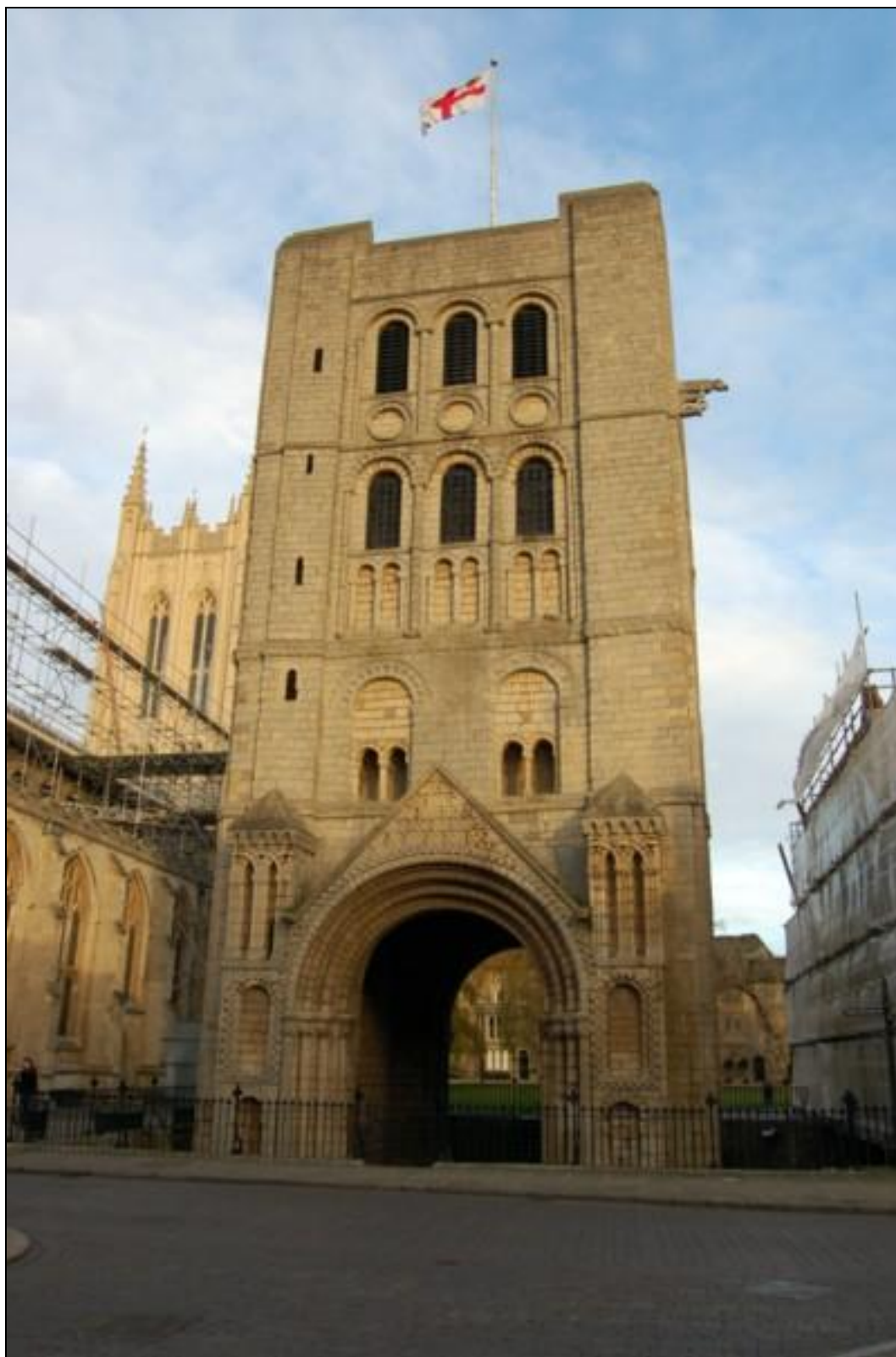
Figure 5.14 The Norman or St James's Tower, photographed from the west. The original ground surface was 2m (8ft) below the modern road.
