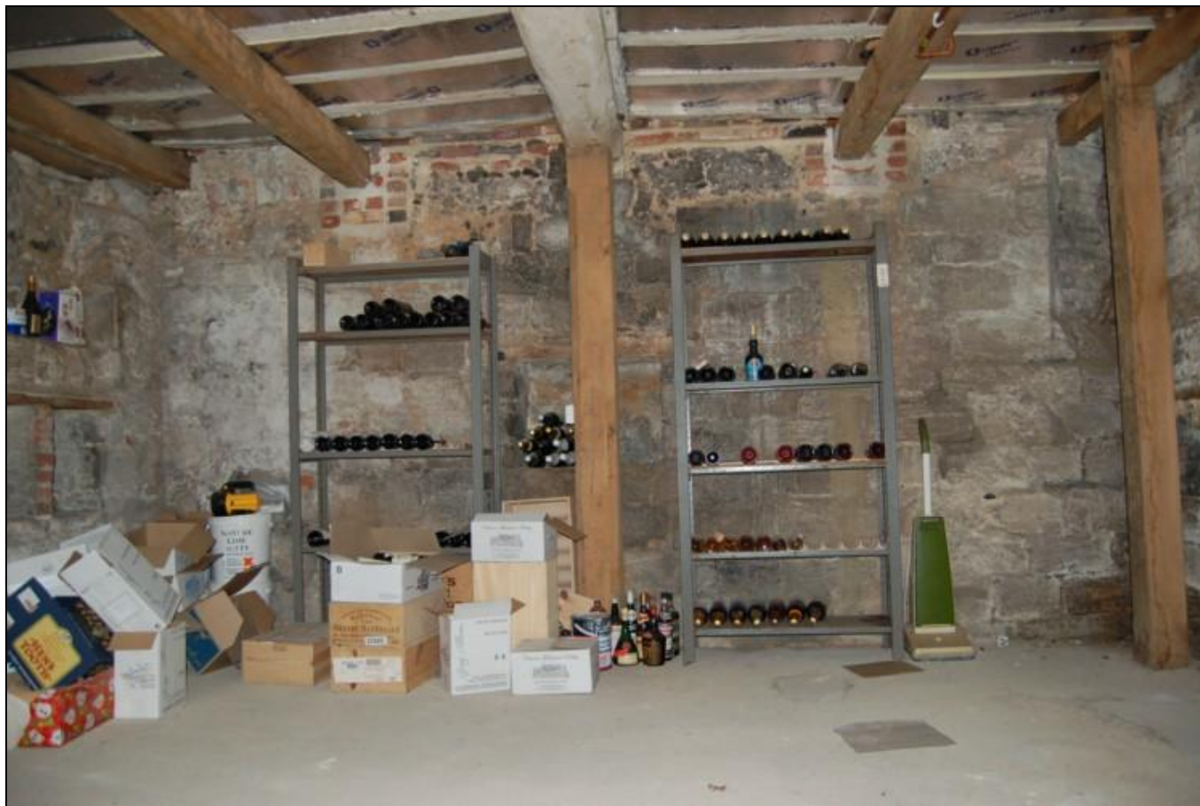
Figure 6.48 The north wall of the cellar of 3, Chequer Square. This looks to be older than the other walls of the cellar, which are constructed from flint rubble. At the eastern end (right hand side) there is a chamfered corner.
