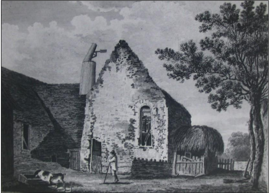
Figure 4.15 St Botolph's Chapel, Southgate Street, before 1804, included as a plate in a collection of manuscript notes (Yates SROB P755/33). This building stood on a plot to the south of the River Linnet (see Figure 4.14 for location).
