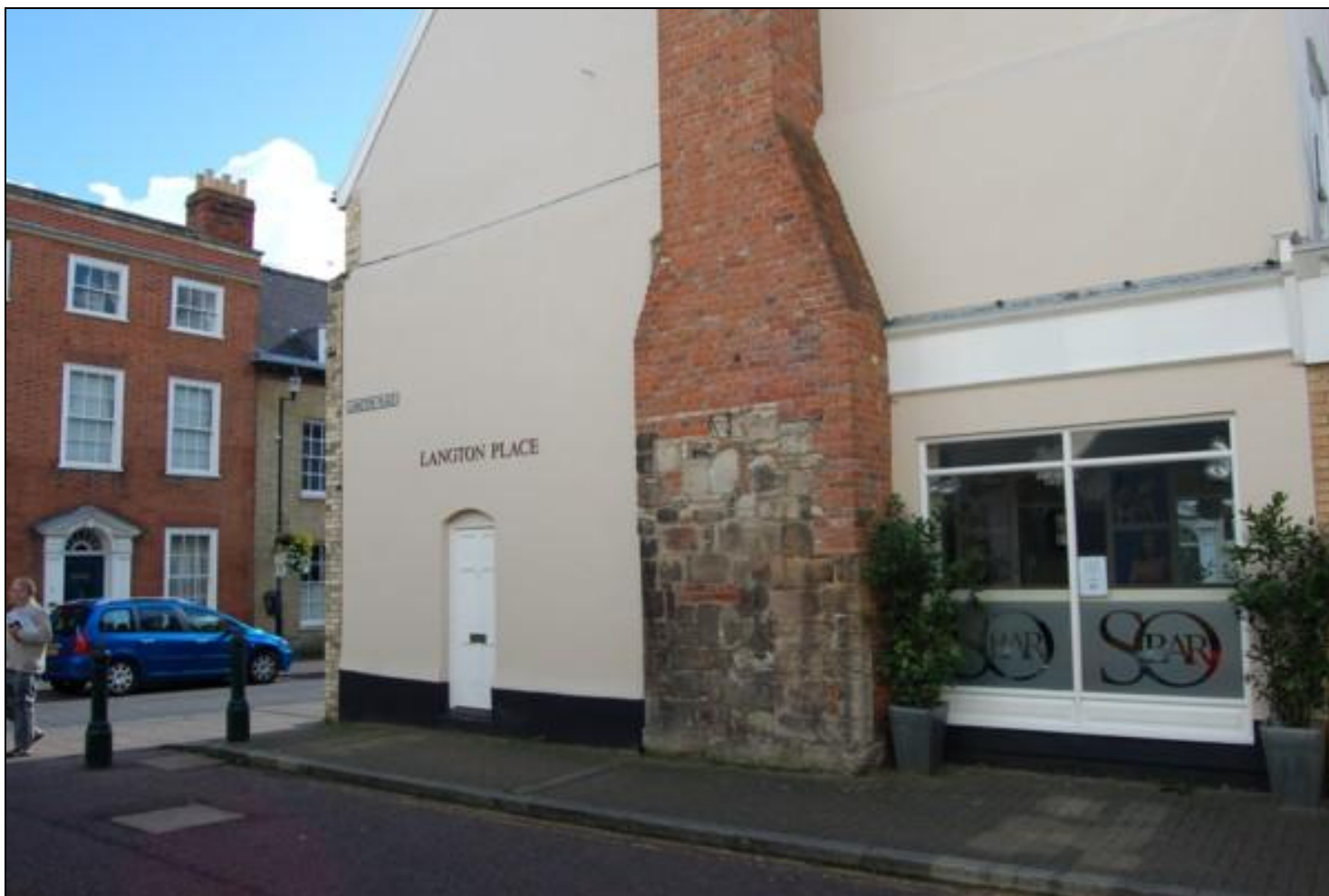
Figure 6.33 Fragment of stonework, 21 Hatter Street. The base of the feature appears to be in situ .
