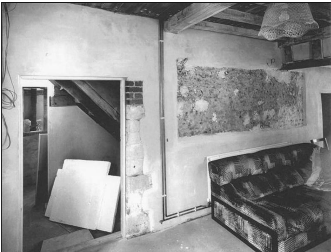
Figure 6.40 The medieval stone wall within 18 Bridewell Lane, photographed in 1989. Figure 6.40a is taken from the southwest and shows that the wall runs up to first floor height. Figure 6.40b, also from the southwest, shows the quoining that probably marks a former doorway. (Both RCHME 89/1404 ©NMR).
