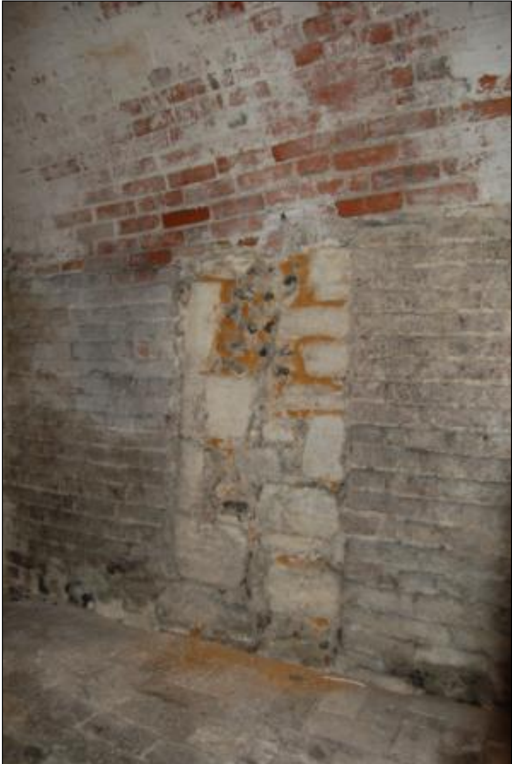
Figure 6.35 Feature in the west wall (towards the street) of 87 Whiting Street. If this is in situ it may be the remains of an arcade or an opening towards the street. The base of the feature is 0.67m wide.
