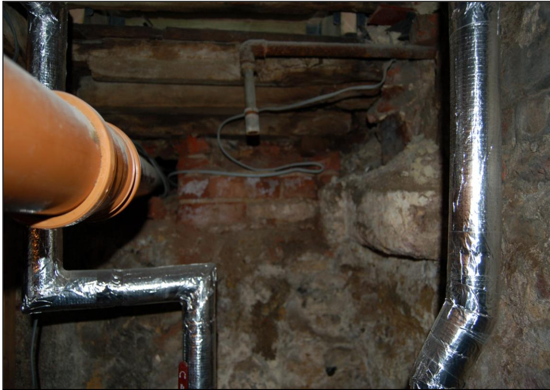
Figure 6.28: Remains of a stair visible in the north-east corner of the cellar beneath 7, Athenaum Lane.
