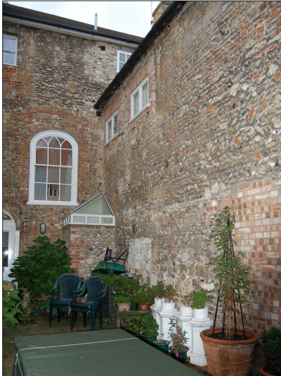
Figure 3.8 The rear wall of 8, Hatter Street, facing west. There are several phases present in the fabric of the wall, and the picture illustrates the re-use of medieval stone. Flint and worked limestone are included in patches of rubble walling, which also incorporate broken brick. Many 18 th and 19 th century walls in the town look similar, and are undoubtedly comprised of post-dissolution monastic rubble. In this case, however, it is possible that the stone was originally used on this site. There are the remains of medieval stonework in the cellar (probably 14 th –century), and, as discussed in Section 6.5.4, an early roof structure remains in situ .
