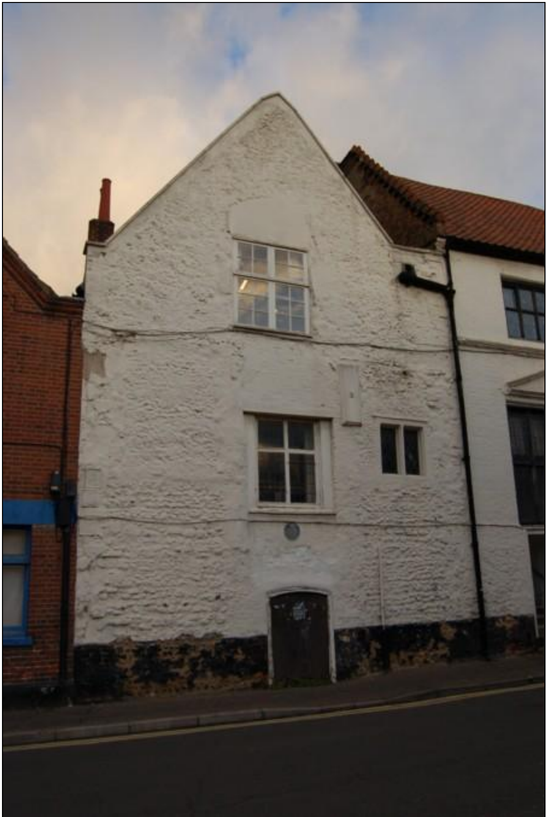
Figure 2.1 Increasingly throughout the 12 th -century, stone houses were built in European towns. Their remains are sometimes still extant. The northern wing of Jurnet's House (or The Music House), King Street, Norwich, here photographed from the west, was originally built in the 12 th century.
